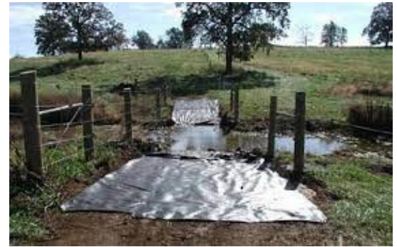
(Photo 1) Photo Credit: AEN-101: Stream Crossings for
